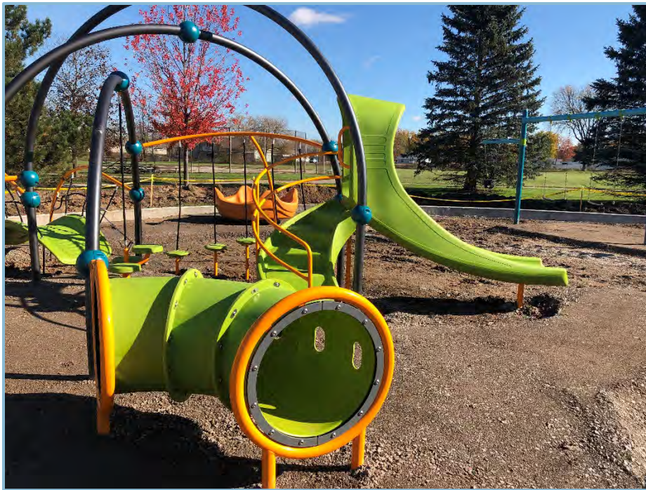
Construction photo of recent playground addition at Williams Township Park.
